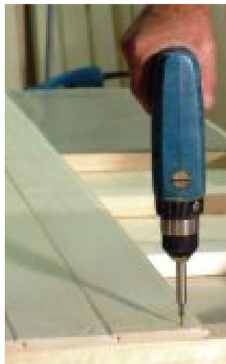
Each board is being double screwed at each end with non-corrosive steel screws.
